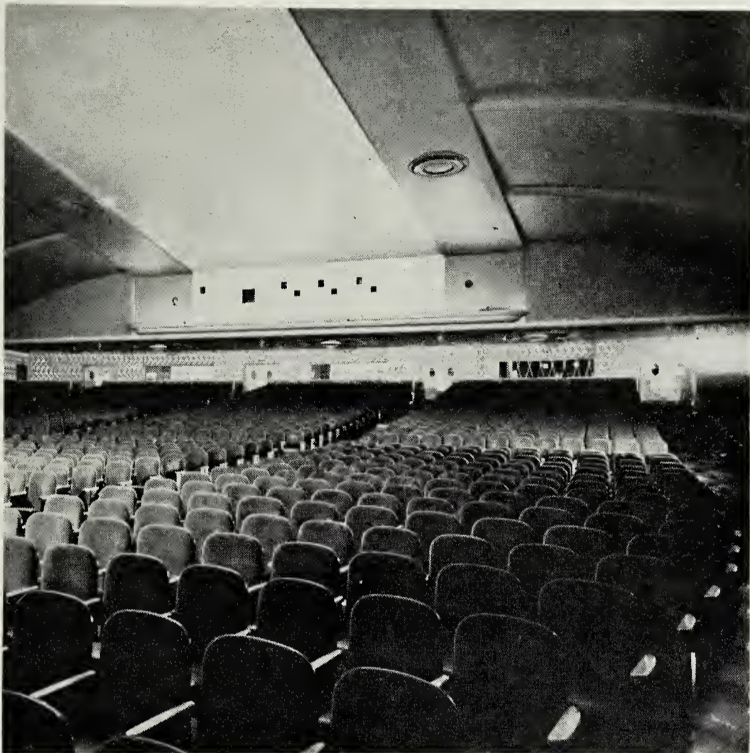
The annoying problem of standees disturbing seated patrons was eliminated at the City Line, Philadelphia, by the construction of a wall between the standee space and the auditorium. The last row of seats is placed five feet away from the wall.
